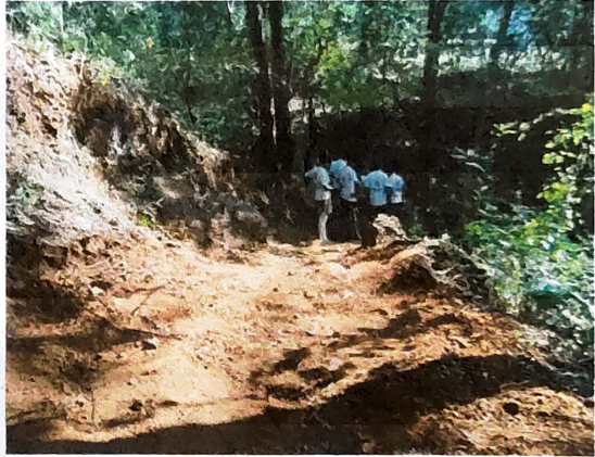
Rough road construction
